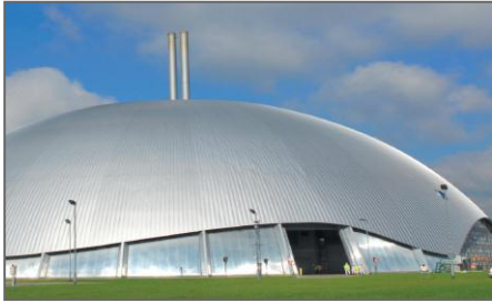
Integrated waste management contracts based on material and energy recovery
